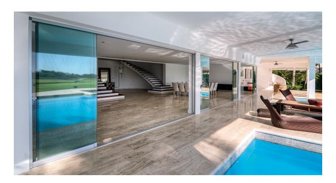
Seeglass-run is an ideal glass system solution for places where you do not want to invade the inside space, like restaurants, terraces and commercial spaces. This system offers the possibility of moving panels, horizontally to one or both sides. Thanks to specially designed panel caps, when the first panel is opened or closed it pulls the rest of the panels so they can be moved as a unit.
